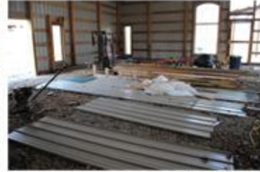
Metal still waiting installation
