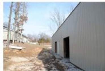
Looking towards the front of new structure
