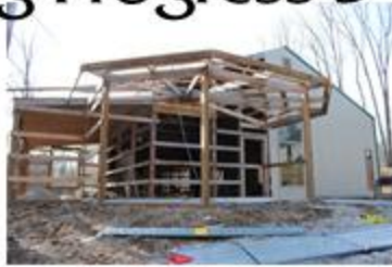
Front entry roof framed for metal
