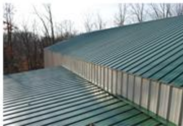
Roof view to rear of building
